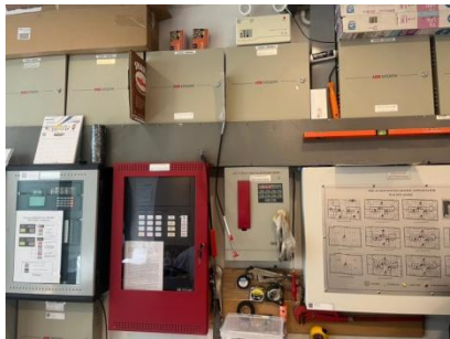
Graphic Annunciator Fire Alarm
